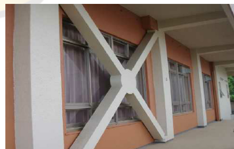
Figure 2: RC Building retrofitted by steel bracing
